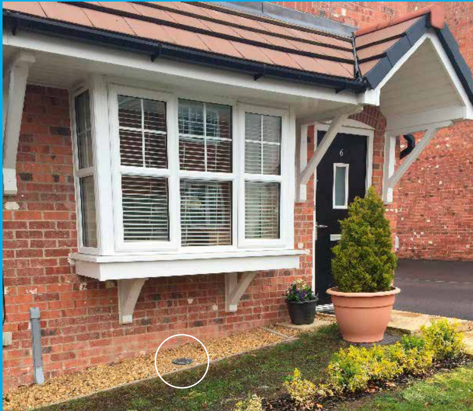
Meter chamber installed within 1m of the front face of the property
