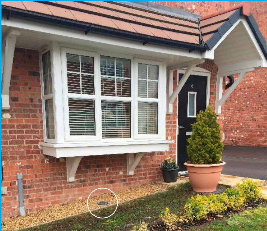
Meter chamber installed within 1m of the front face of the property
