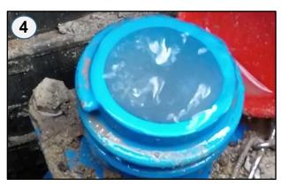
FLUSH THE HYDRANT OF ANY DEBRIS UNTIL IT RUNS CLEAR, THEN TURN THE HYDRANT OFF **SLOWLY**
