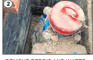
REMOVE DEBRIS AND WATER FROM HYDRANT PIT USING APPROPRIATE TOOLS. **DO NOT PUT HANDS INTO HYDRANT PIT**
