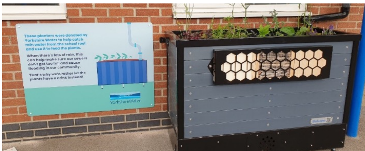
A SuDS planter (Sustainable Drainage System planter) we installed at Cayton Bay School, in Cayton, Scarborough.
