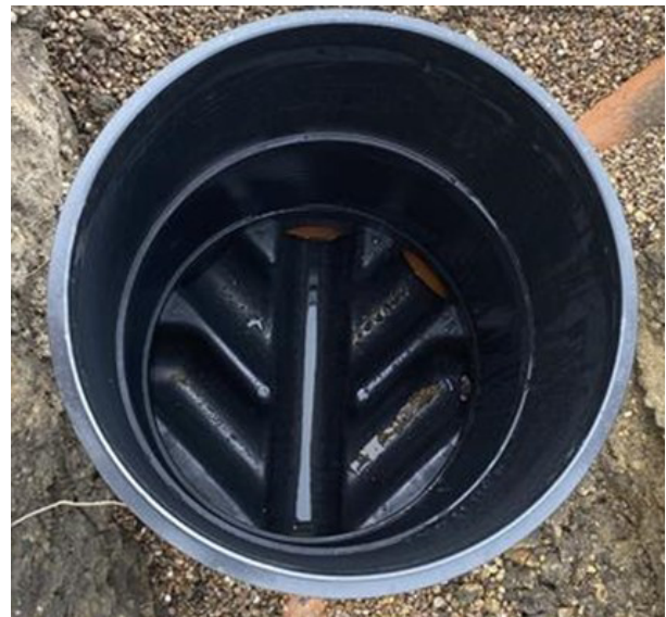
Connection into a new demarcation chamber
