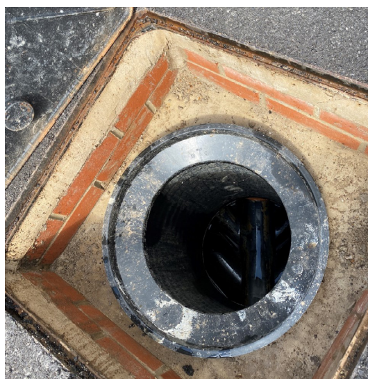
Brickwork above a polypropylene inspection chamber (PPIC)
