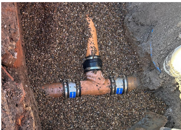
Junction connection with pea gravel
