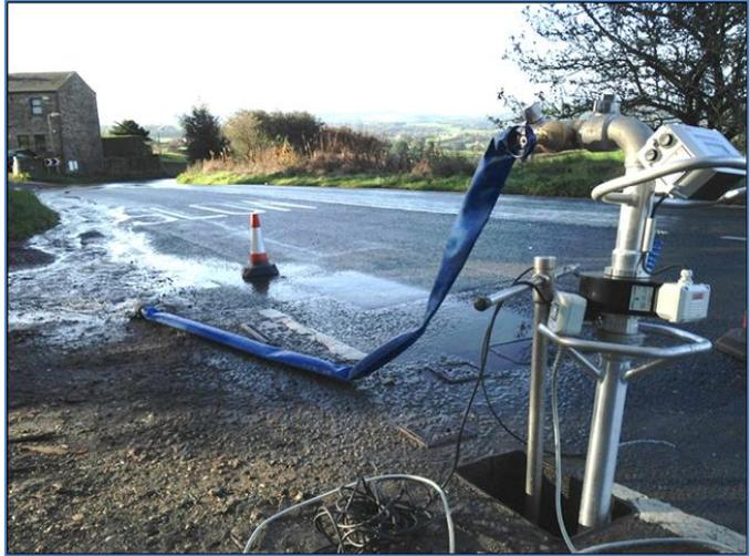
Figure. 36: Networks flushing showing flow and quality monitoring on standpipe.
