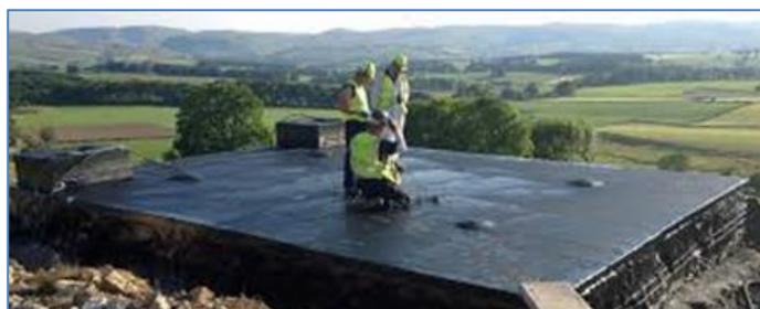
Figure. 38: Service Reservoir roof membrane installation.
