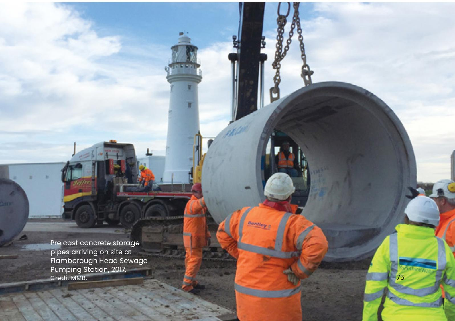
Pre cast concrete storage pipes arriving on site at Flamborough Head Sewage Pumping Station, 2017. Credit MMB.
