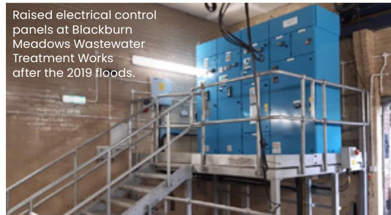
Raised electrical control panels at Blackburn Meadows Wastewater Treatment Works after the 2019 floods.
