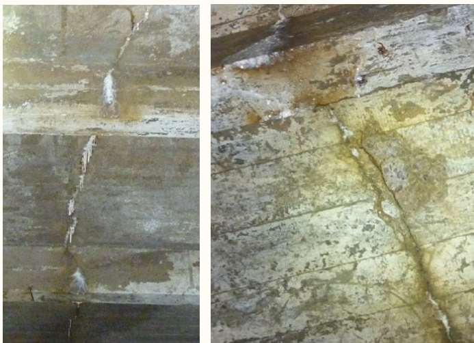
Figure 8-6 showing historic cracking to the roof structure. This shows any damage to the loose laid membrane on the exterior roof could lead to multiple points of ingress.
