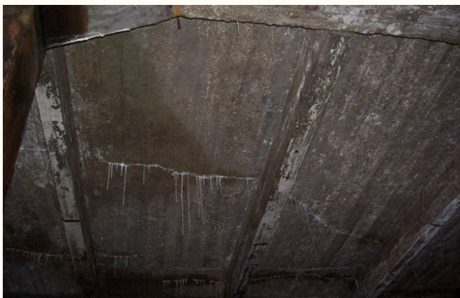
Figure 8-4 Internal cracking widespread throughout the structure roof.
