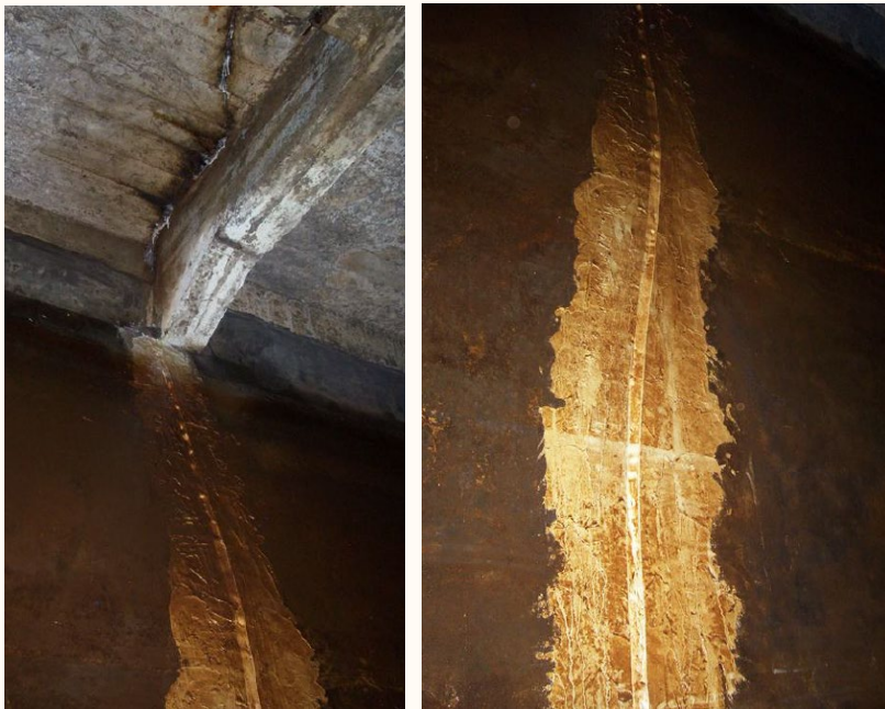
Figure 8-5 Demonstrates extensive over-banding repairs on the longitudinal wall sections
