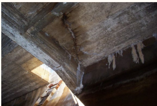
Figure 8-3 Showing Internal cracking and historic repairs on the structure roof.
