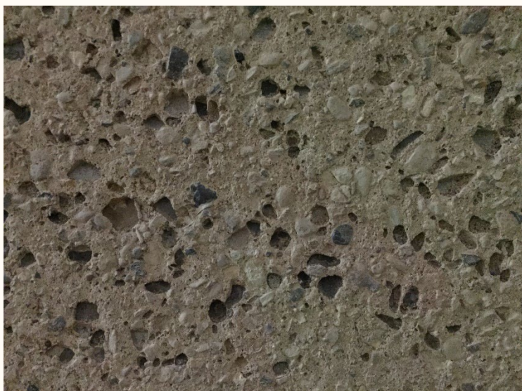
Figure 8-7 RGF Concrete degradation at Loftsome WTW
