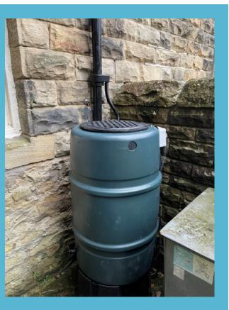
which water enters our wastewater network during storm events. These slowly drain down in advance of forecasted heavy rainfall, giving more capacity to hold back rainwater and reducing the risk of the wastewater system becoming overwhelmed.
