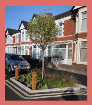
SuDS offer a more natural alternative to rainwater flowing directly into the sewers, which are sometimes unable to cope with extremely heavy rainfall. Instead, rainwater is transported into green areas to be soaked up by plants and trees or stored in ponds and drained away more slowly to a watercourse or the sewer.
