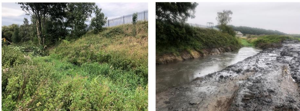
Figure 120: Lundwood ditch clearance, before and after
