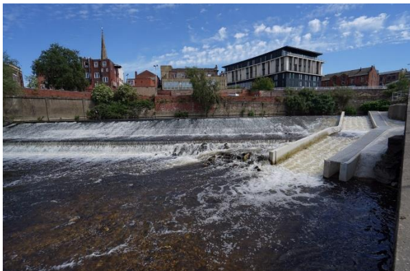
Figure 118: Installed fish pass at Masborough
