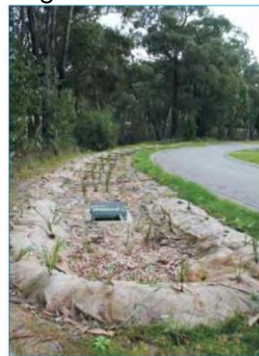
Figure 1 A newly installed retrofit rain garden (courtesy Darren Bos)
