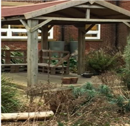
Figure 119: Rainwater harvesting installation within the community
