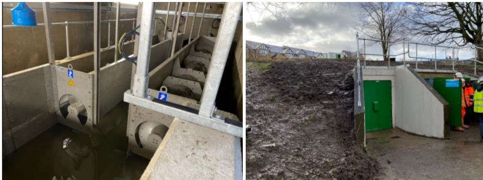
Figure 18: Upgraded screens and panel at Rivadale View Storm Overflow
