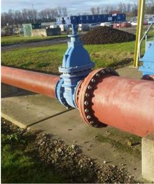
Figure 3 - Tie-in feeding the incinerator compound Treated Water Storage Tank.
