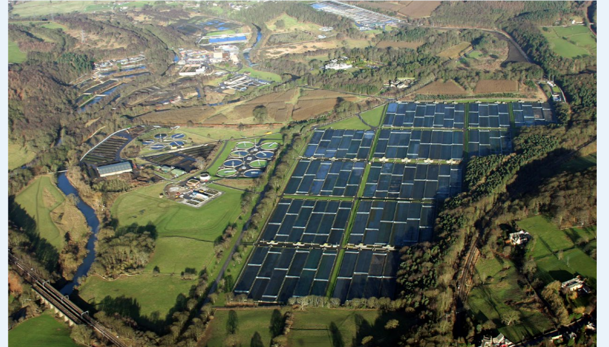
Aerial view of Esholt wastewater treatment works in Bradford
