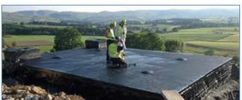
Figure. 38: Service Reservoir roof membrane installation.
