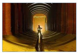
Figure. 37: SR emptied for inspection and cleaning.
