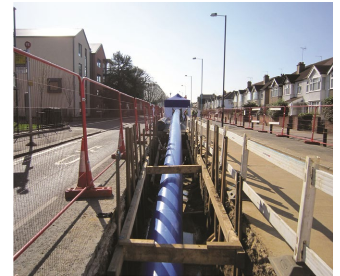
Water pipe replacement
