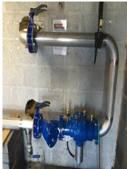
Figure 17: RPZ valve installation
