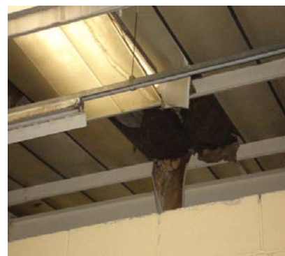
Figure 22 - Depot roof – AMP5 replacement
